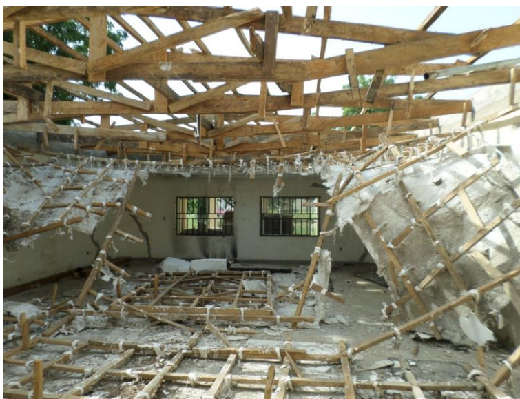
Picture of the secretariat building in Mafa LGA before rehabilitation
