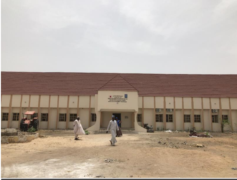
Picture of the secretariat building in Mafa LGA rehabilitated
